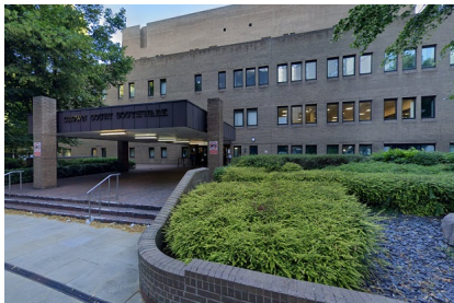
Crown Court Southwark, 1 English Grounds London UK
